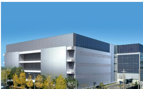
Main data centers in the Tokyo area
